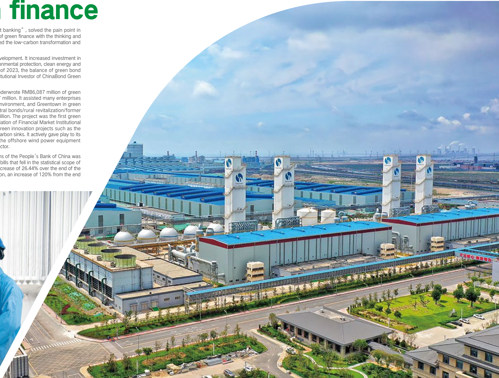
PSBC’s green loans are helping enterprises save energy and reduce resource consumption.
