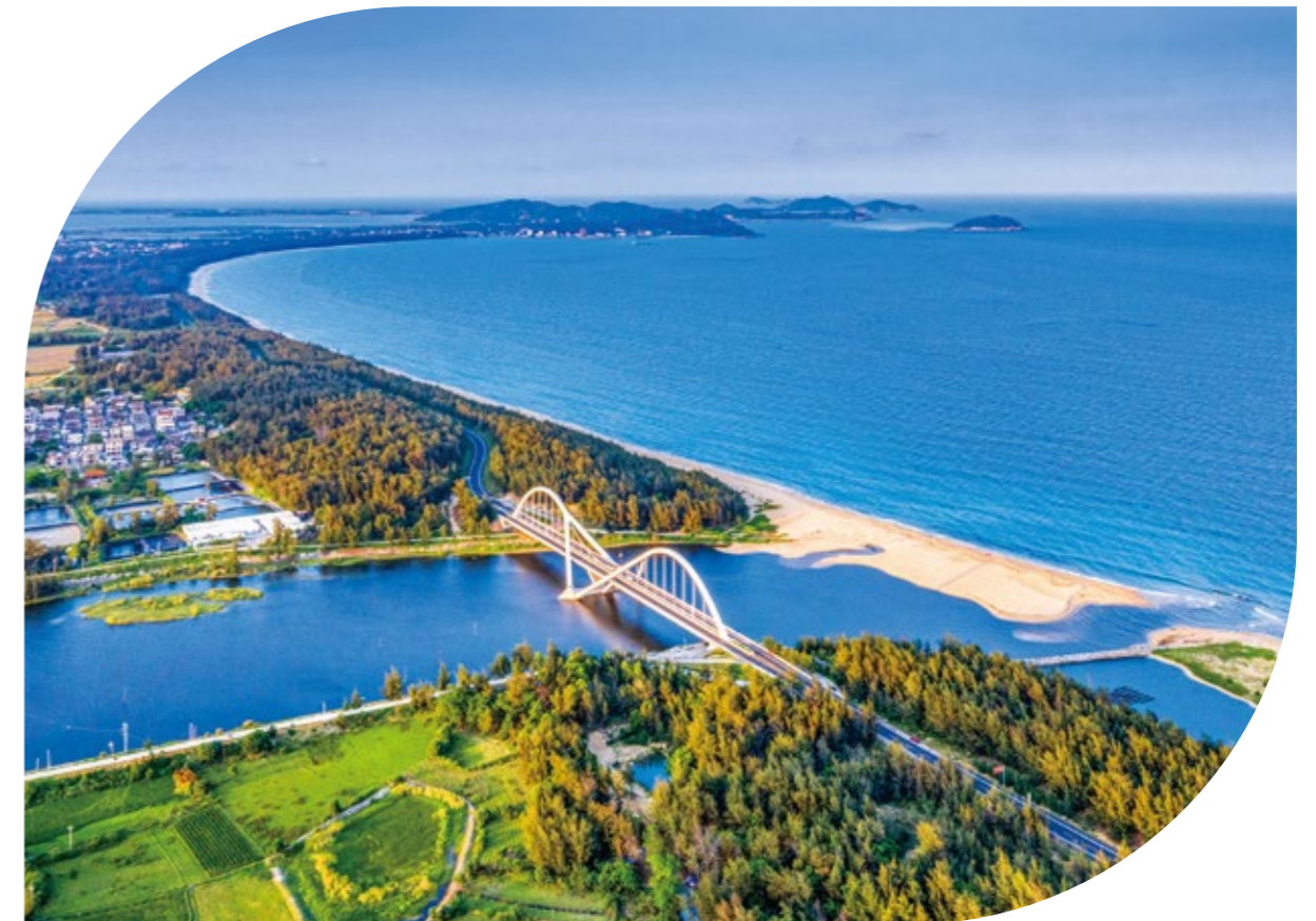
PSBC extended credit for the construction of Hainan Island Ring Road.
